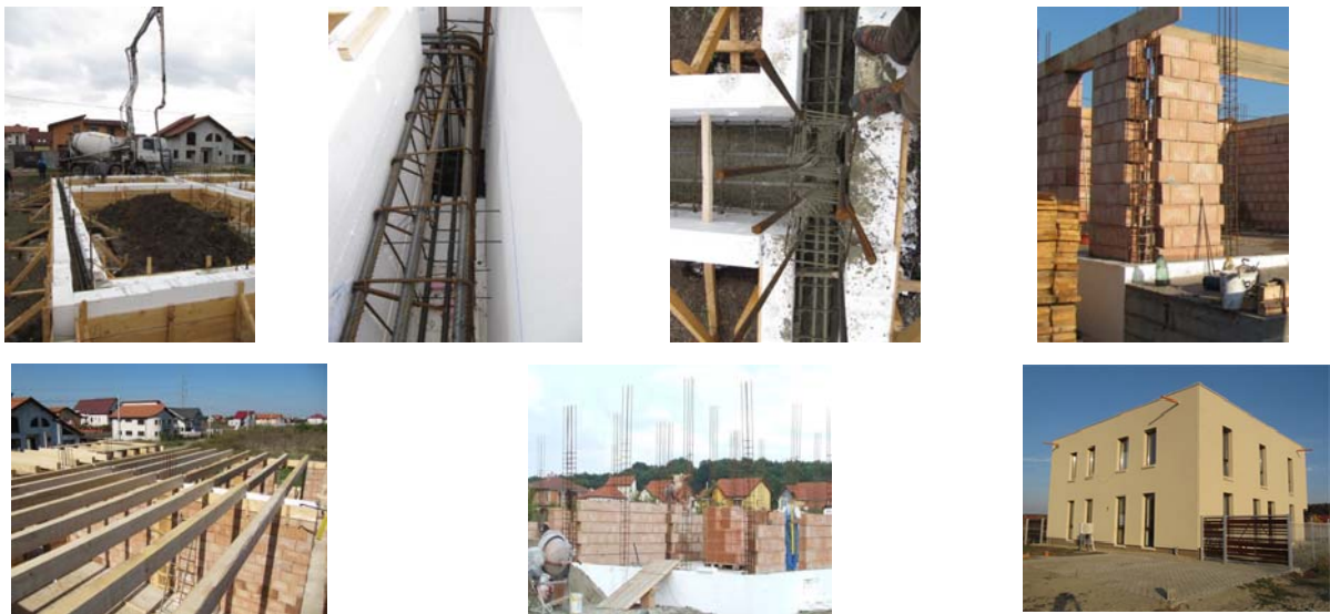
Fig. 3. Pictures from the construction site of the residential house
