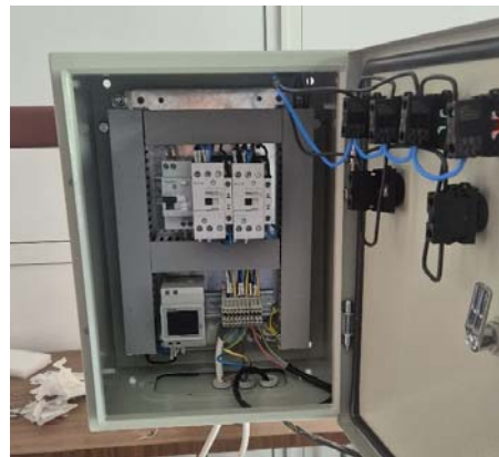
Figure 6 Control and Measurement Electrical Panel
