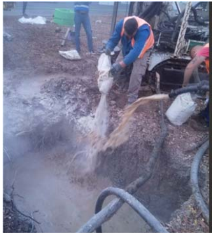
Figure 3-3. Bentonite and water mixture for borehole wall stabilization
