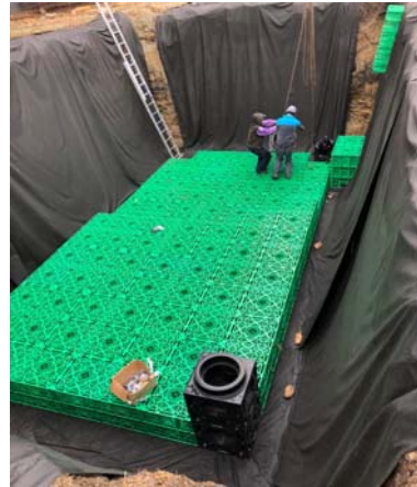
Fig. 6. Details from the tank assembly stage
