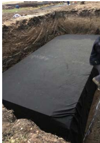
Fig. 8. Covering the tank with geomembrane
