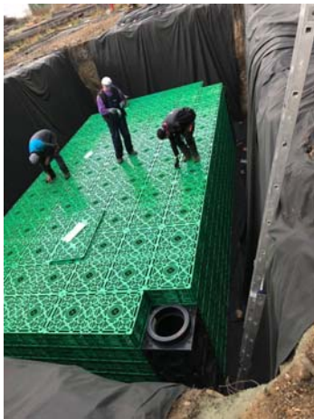
Fig. 7. Preparation for geomembrane coating
