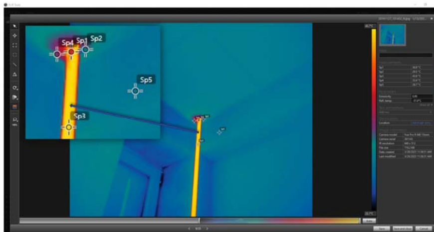
Fig. 7. The pipe entering point from the office' ceiling
