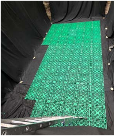
Fig. 5. Geomembrane preparation and tank bottom plate installation stage
