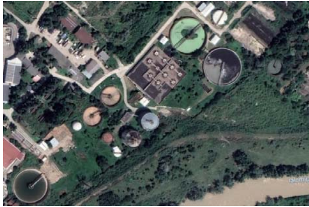
Figure 3 – Slobozia WWTP (Google Earth)
