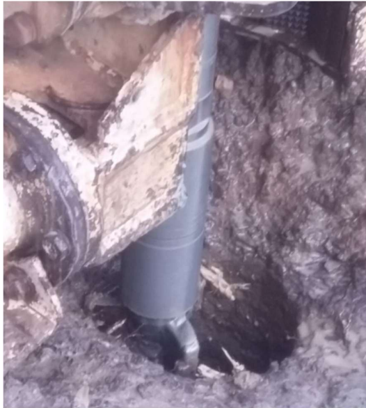
Figure 3-2 Drilling head 160 mm
