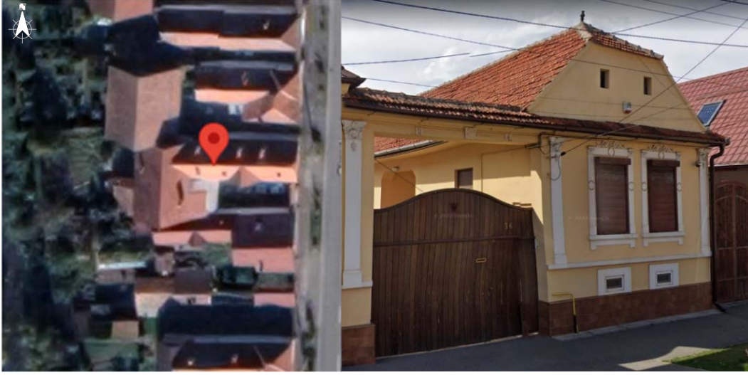
Figure 2. The investigated house.
