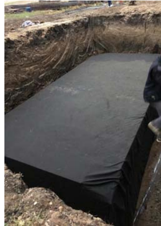
Fig. 8. Covering the tank with geomembrane
