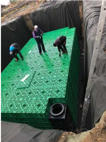
Fig. 7. Preparation for geomembrane coating
