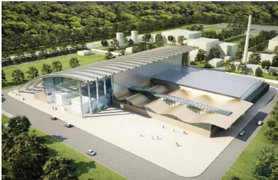
Figure 5 – ELI-NP Building in Magurele, Romania, supplied by more than 1000 BHE, impression of Hachiko (2011)
