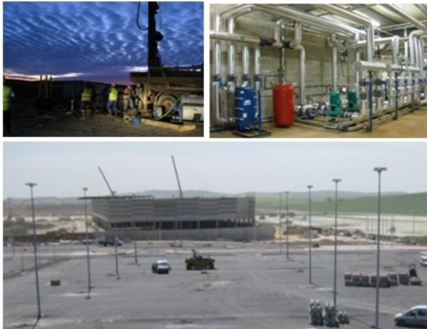
Figure 6 - Furniture retail building in Jerez de la Frontera, Spain, using GSHP predominately for cooling.
